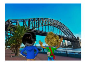
Coathanger, was officially opened on 19 March 1932. In the same year, 96 steam trains were used to test how much weight the Bridge could take. Today, eight lanes of traffic and two rail lines cross the bridge.
